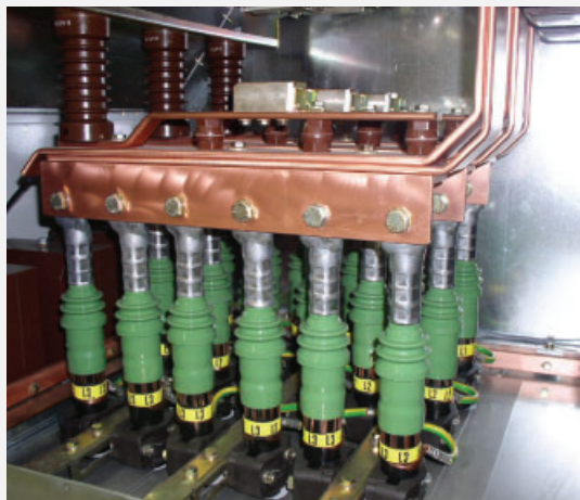
Panel type AMC9-12/2500-2500/31-L cable connection area with 6x1x500mm 2 per phase and capacitive insulators
