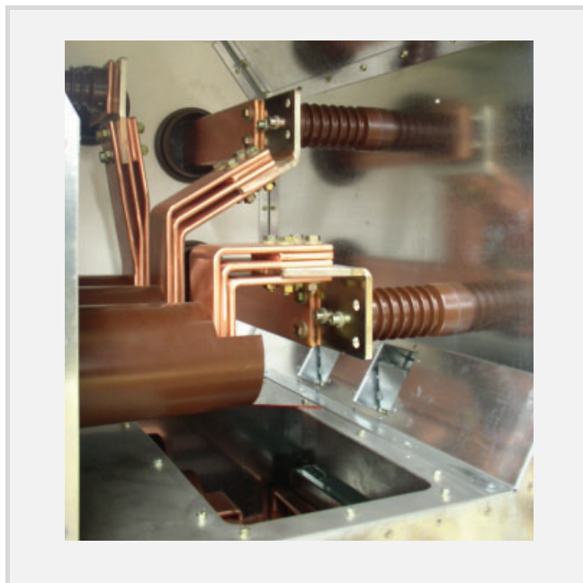
Busbar compartment with capacitive insulators
